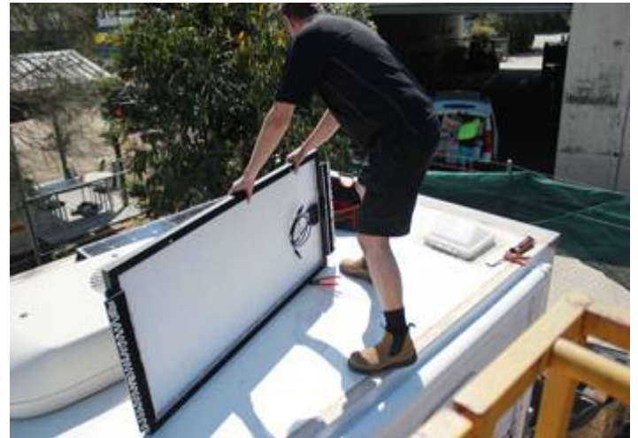
4. Place solar panels to the roof of caravan.
